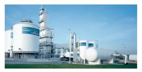
For the industrial production of high purity nitrogen, oxygen, argon and other air gases, the individual air components are separated using a thermal process in air separation plants.
