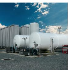
Depending on the quantity, cryogenic air gases are stored in fixed storage tanks with capacities from 5,000 to 50,000 litres.
