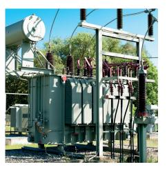
In the local grid, distribution transformers produce the normal voltage of 400/230 Volt.
